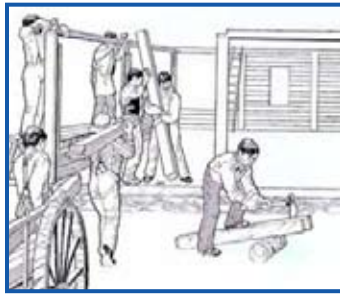
Illustration of Red River frame construction: Parks Canada
