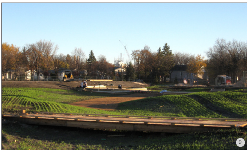
Sculpted berms and rolling hills help direct water flow on site at École St. Avila (Winnipeg, Manitoba).
