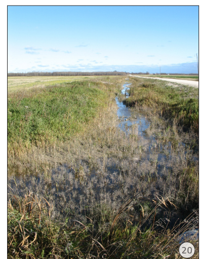
EICD seeded native plants along a freshly excavated ditch in the RM of Woodlands, Manitoba. This bio-retention area helps filter runoff and prevent soil erosion.
