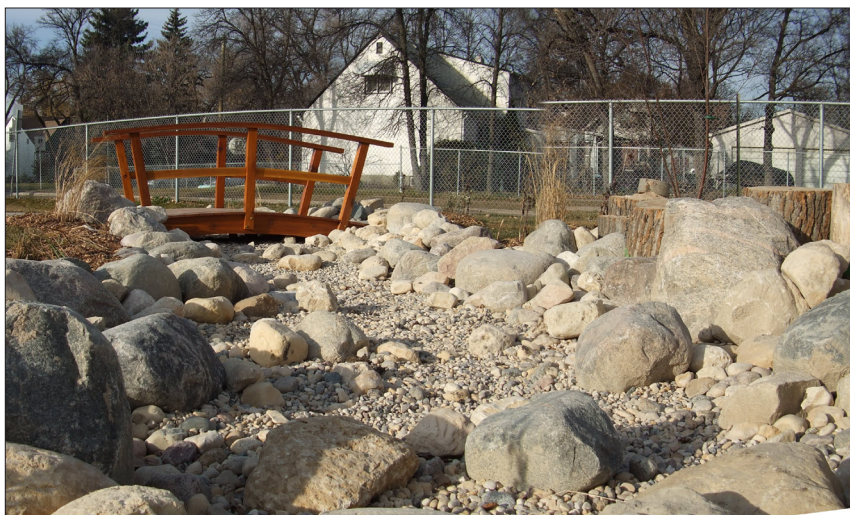
At the Linwood Child Centre, a dry stream (dry swale) complete with a timber bridge helps to facilitate site drainage, while focussing on natural play (Winnipeg, Manitoba).
