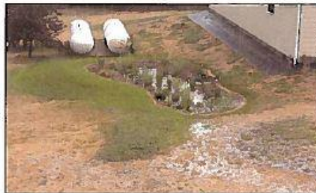
Figure 2. A new rain garden captures roof and yard runoff from a 1/2 inch, 15-minute prairie thunder storm in July. Note the drought stressed yard outside the rain garden.
